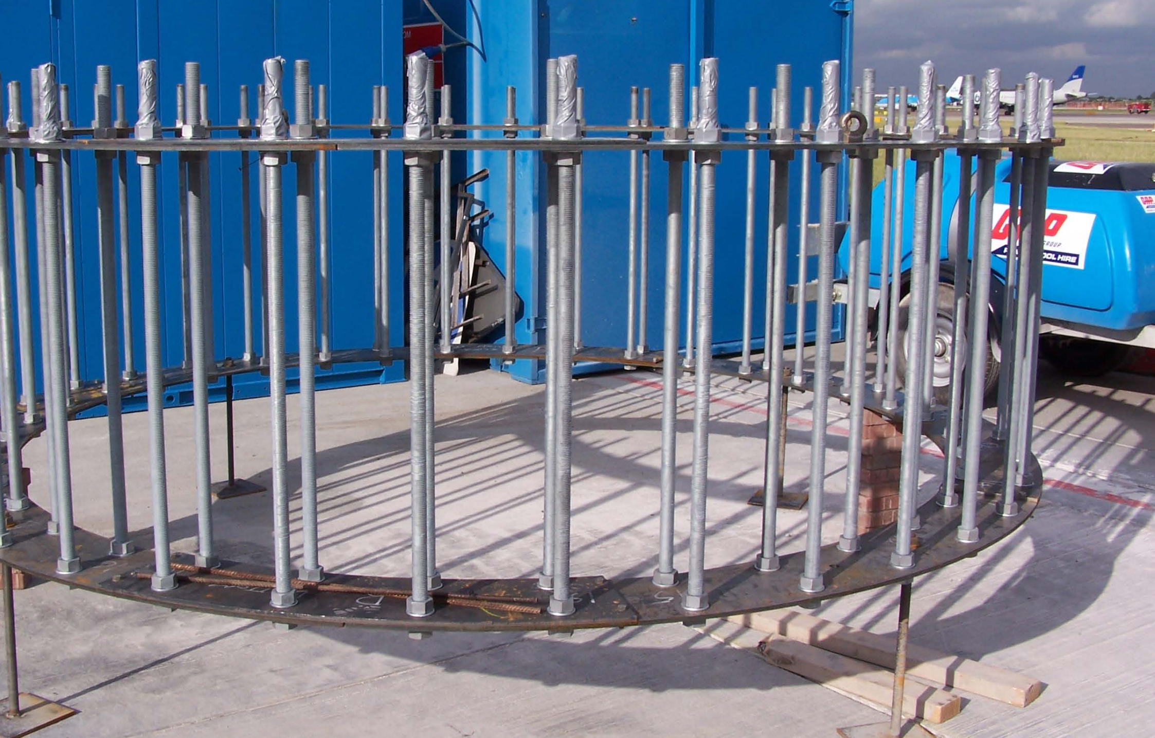
Pre-assembled foundation ring for 25m SMR Monotube Tower at Heathrow Airport, UK
