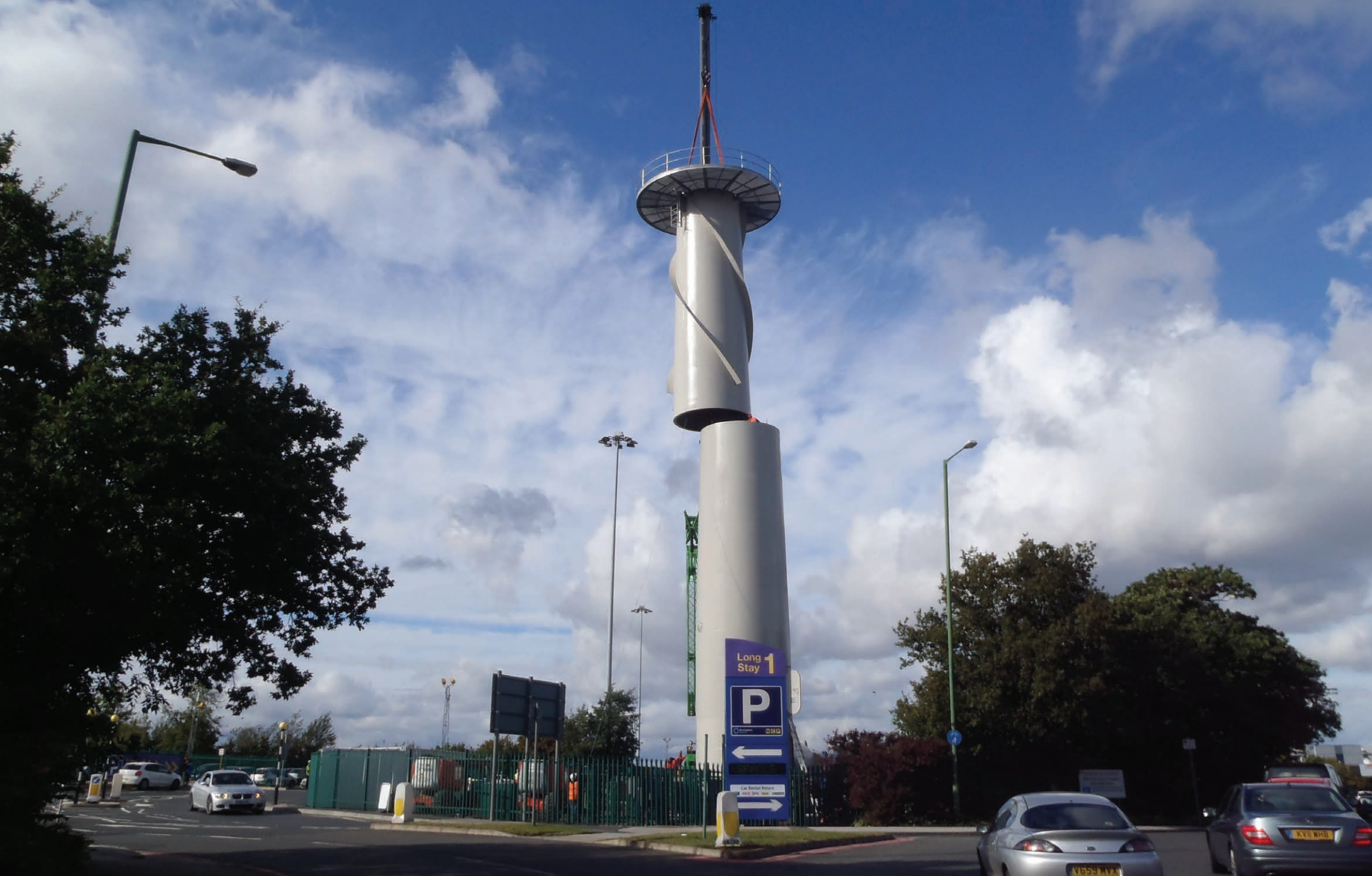
Birmingham Airport, UK 30M PSR Monotube Tower Ideally located to minimise impact on local communities
