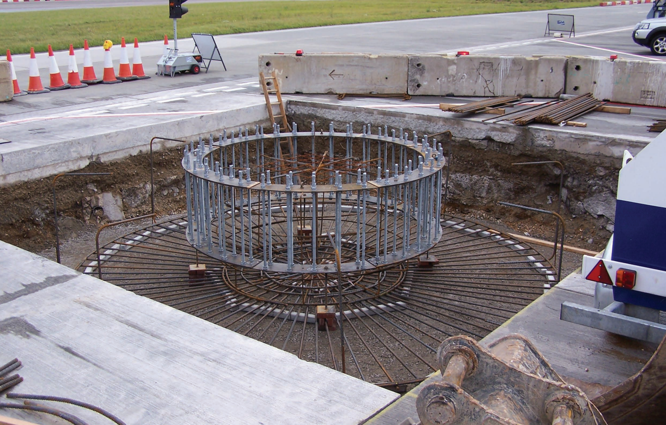
Ground Works for 25M SMR Monotube Tower at Heathrow
