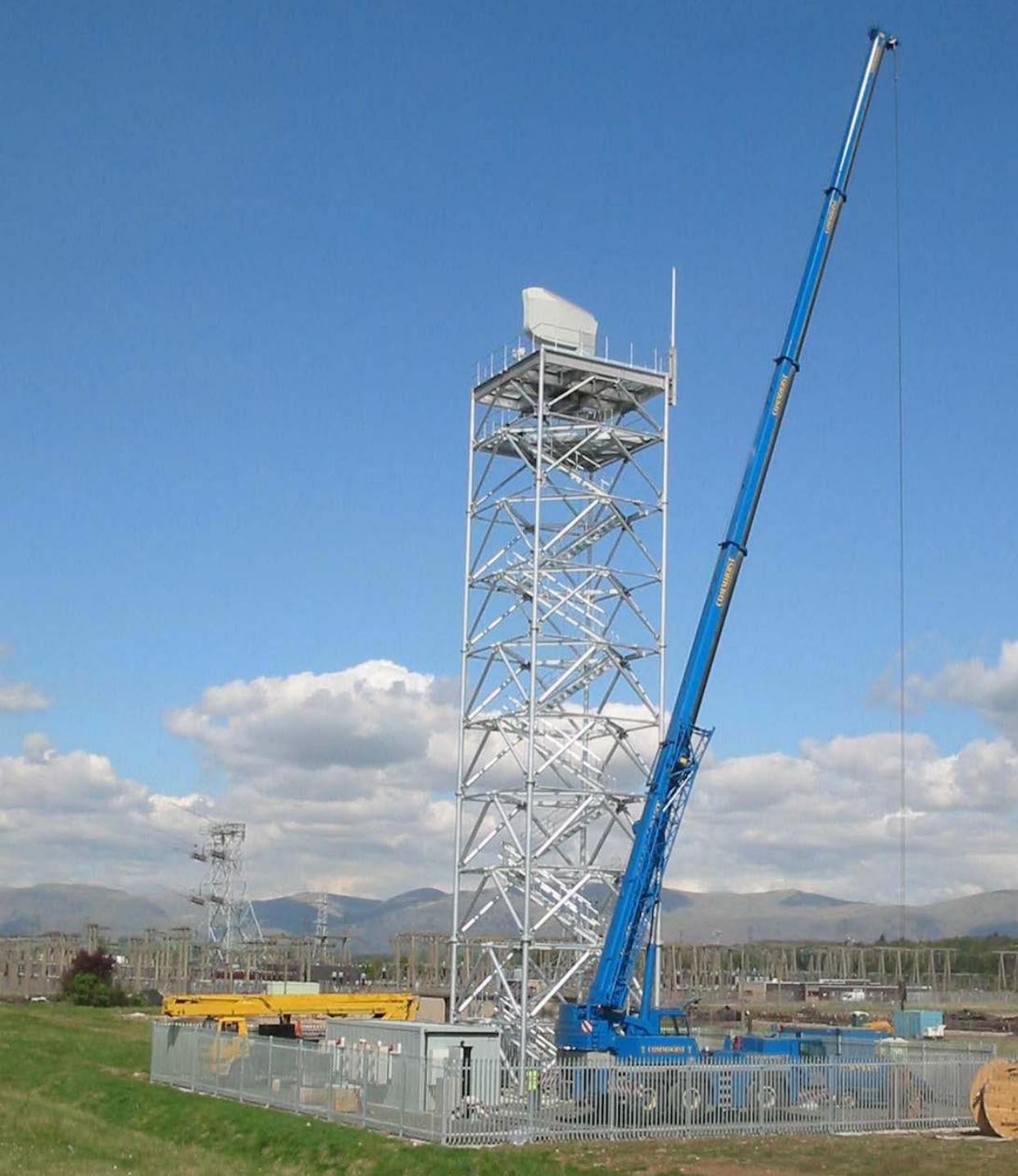
Installation of 30m Galvanised Steel Lattice Tower with integral staircase to top platform
