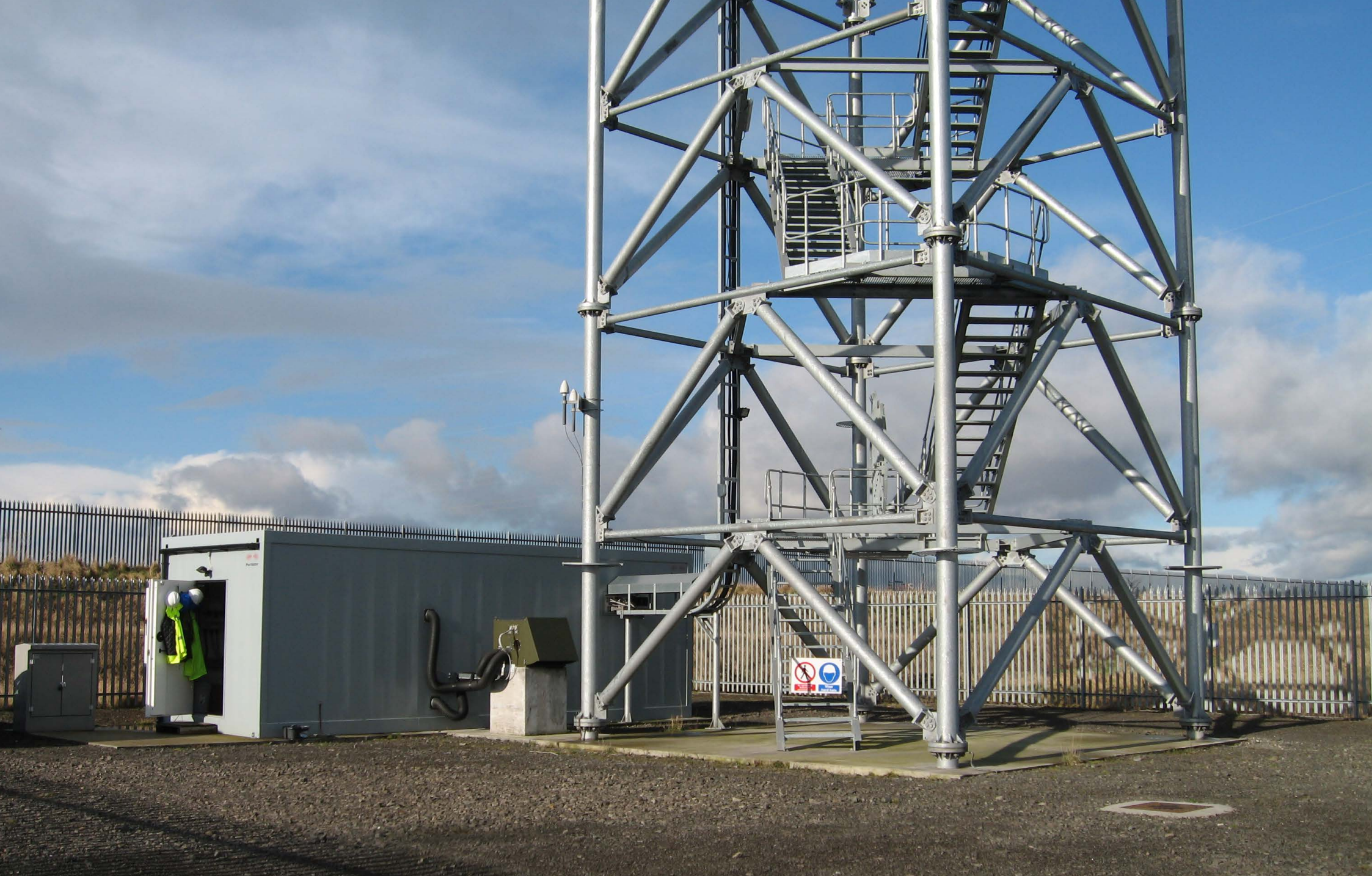
Radar Compound works at Kincardine UK
