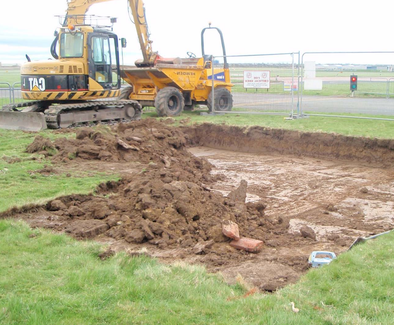
Civil Works at Hawarden Airport, UK.
